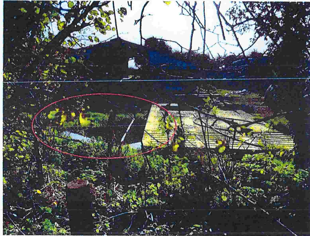
Fig No. 6 Ponding in the area of the proposed soak pit (beside unknown platform not identified in the site layout plan). Photo taken from Brennan property at location in field north of the site.
